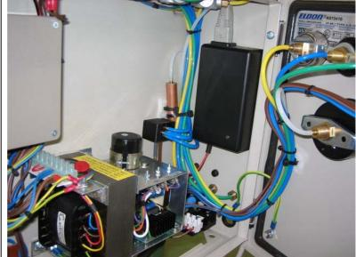
16) Connect the supply for the transformer to the power pack terminals N (Neutral – Blue wire) and 8 (Line – Brown wire). Connect the Yellow/green wire to the earth screw.
