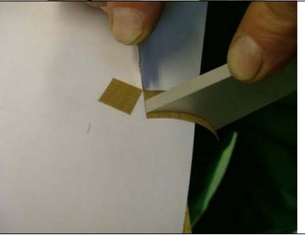
9. Cut the curved edges of the tray ends, using the aluminium as a guide to make a flush cut.
